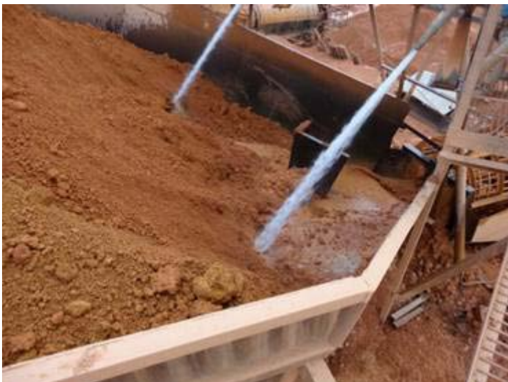
Cargo filtering using high pressure water and sieves
