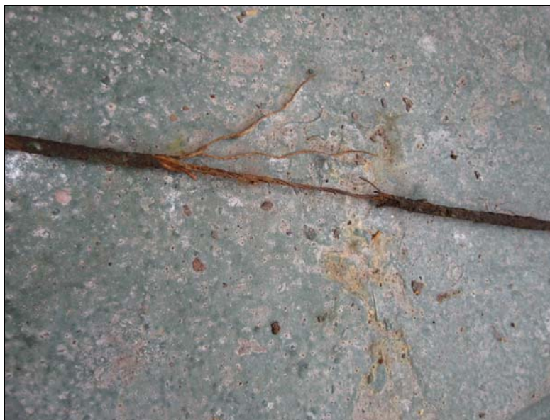
Figure 20: Damage remote control cabler
