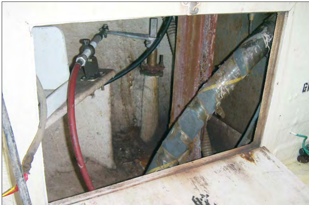
Figure 3: After bulkhead inside the boat with access door open
