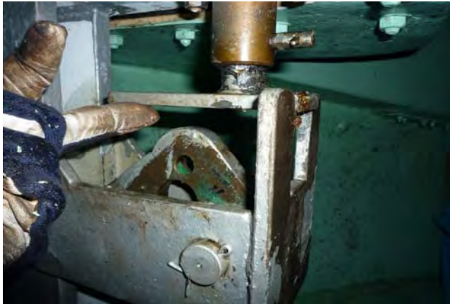
Photo 2 and 3: Under-deck cam plate.
