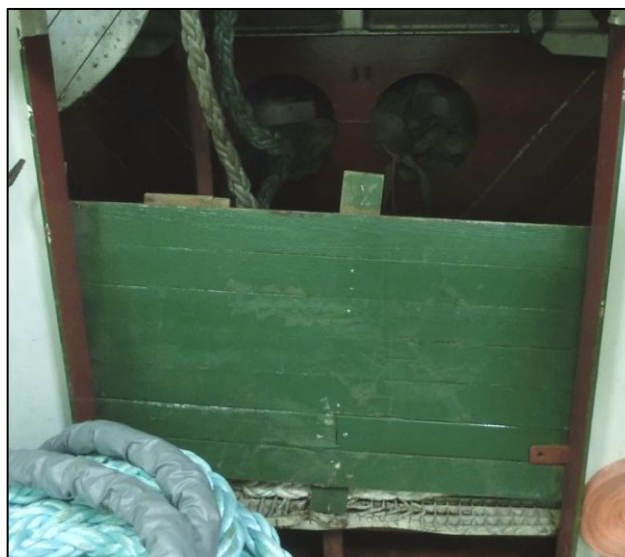
Figure 3: Wooden boards in use to block access
