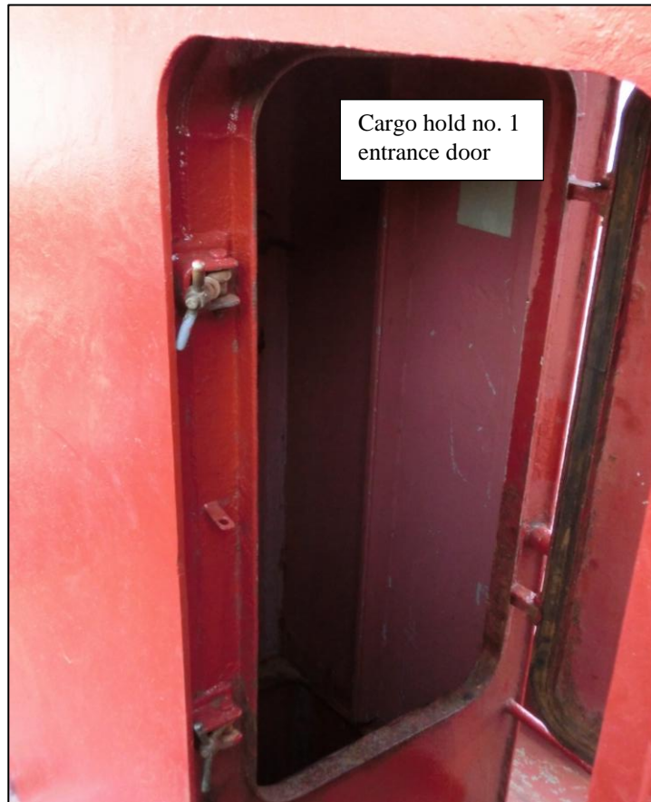
Figure 5: Entrance to cargo hold no. 1
